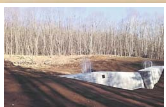
■古仙西沢砂防堰堤 (長坂町小荒間)
